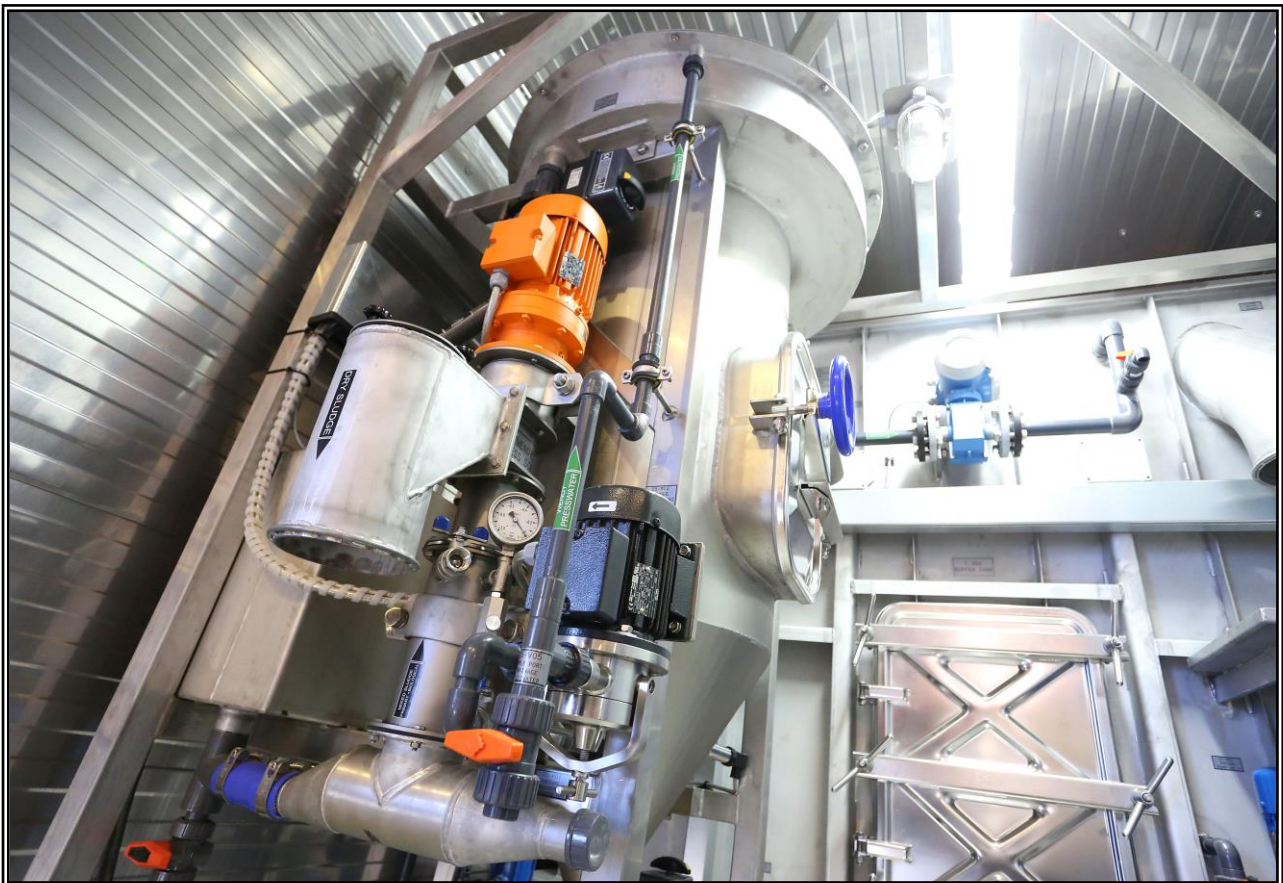
ExSep® as part of Epuramat's Box4Water containerized wastewater treatment plant
