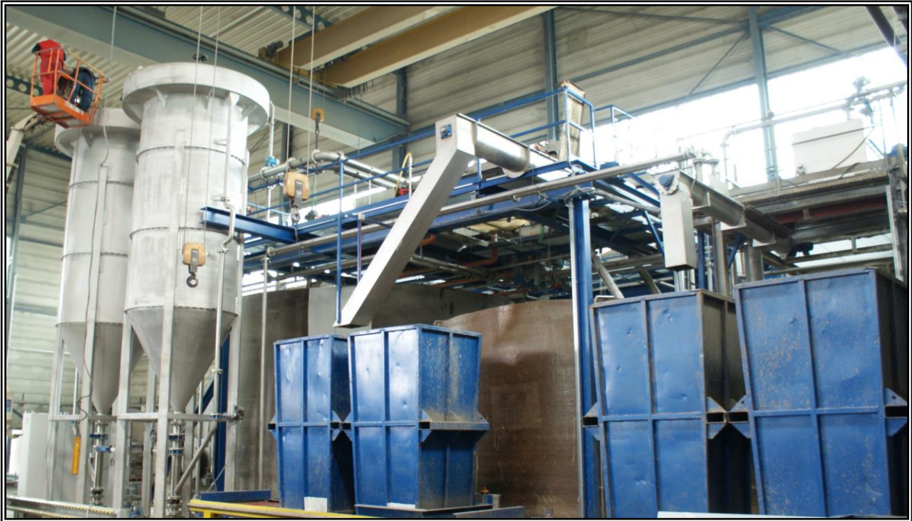
ExSep® system with two ExSep® 2000 for reuse of process water from a soil and plastic recycling company
